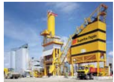
Old asphalt can be recycled.
