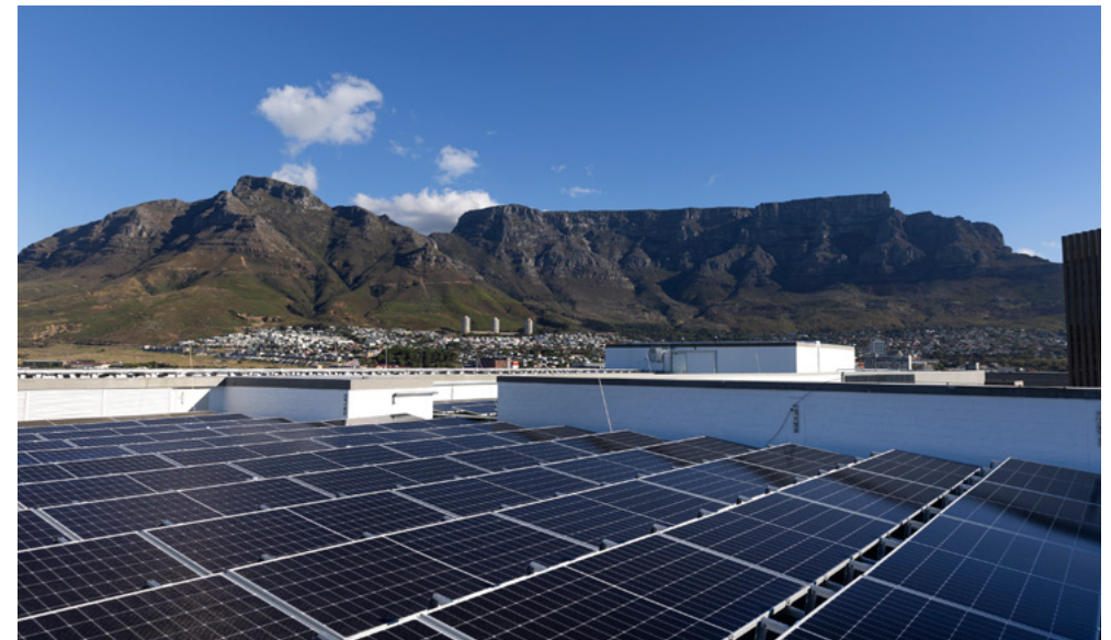
At the SASAII CT Station project, Cape Town, South Africa.
